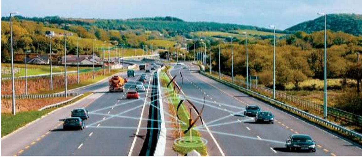
Figure 5. Wind energy on highways (Anonymous, 2024c).
