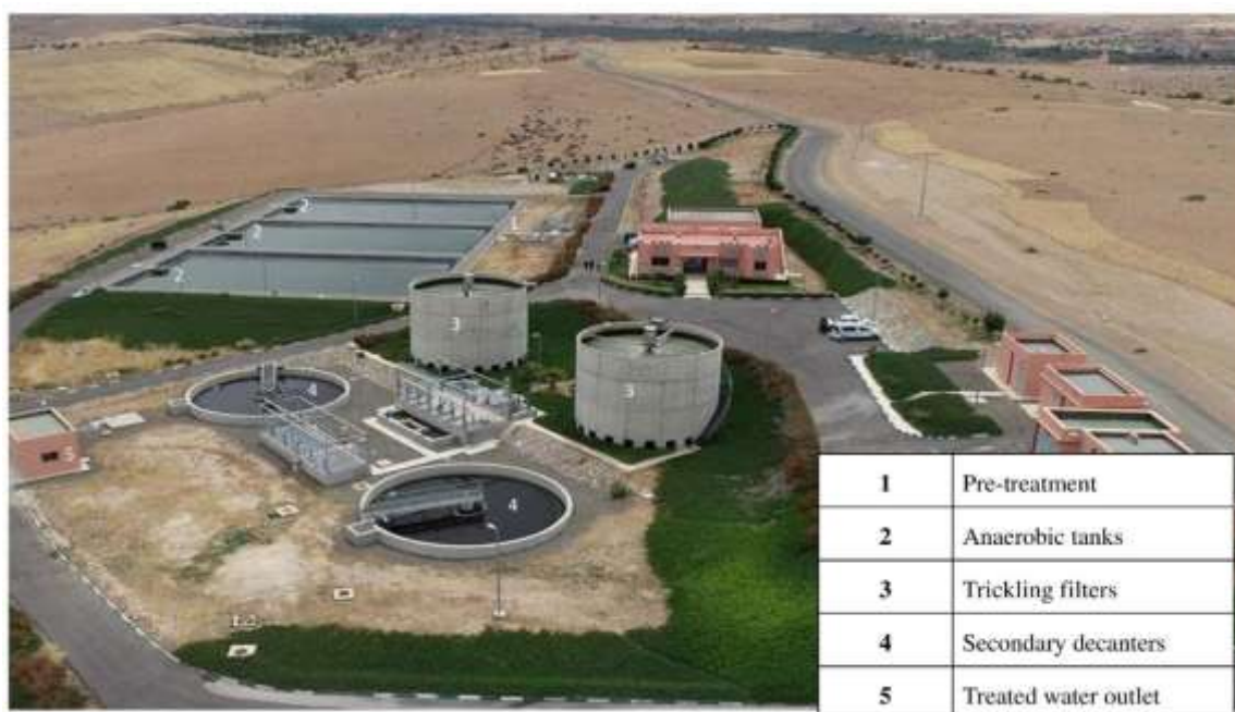
Fig.1. Presentation of the full-scale trickling filter system at Imintanout city (Morocco)
